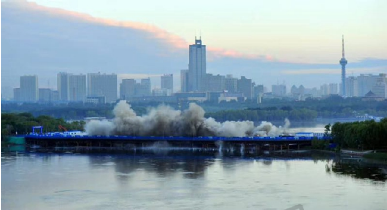
Explosives brought down Nanhu Bridge in Changchun, capital of northeast China's Jilin province, within seconds on June 11, 2017. [Photo by Wan Jigang/chinadaily.com.cn]
