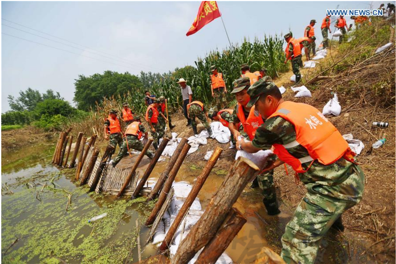
Armed police ram wood piles to reinforce the dyke of Poyang Lake in Jiujiang City, east China's Jiangxi Province, July 11, 2016. (Xinhua)
