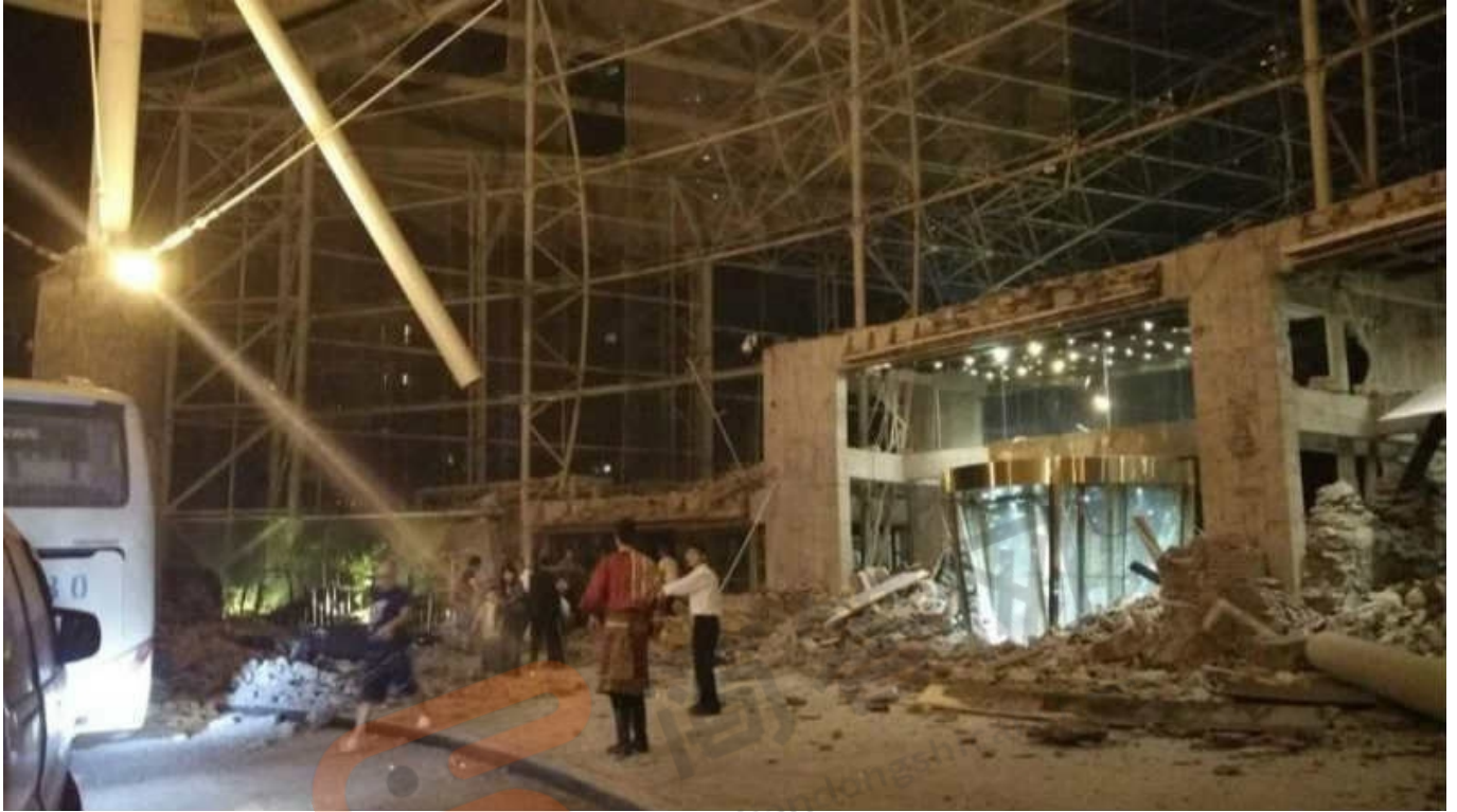
The front gate of a hotel is damaged after the earthquake in Jiuzhaigou County of southwest China's Sichuan Province./Xinhua Photo
