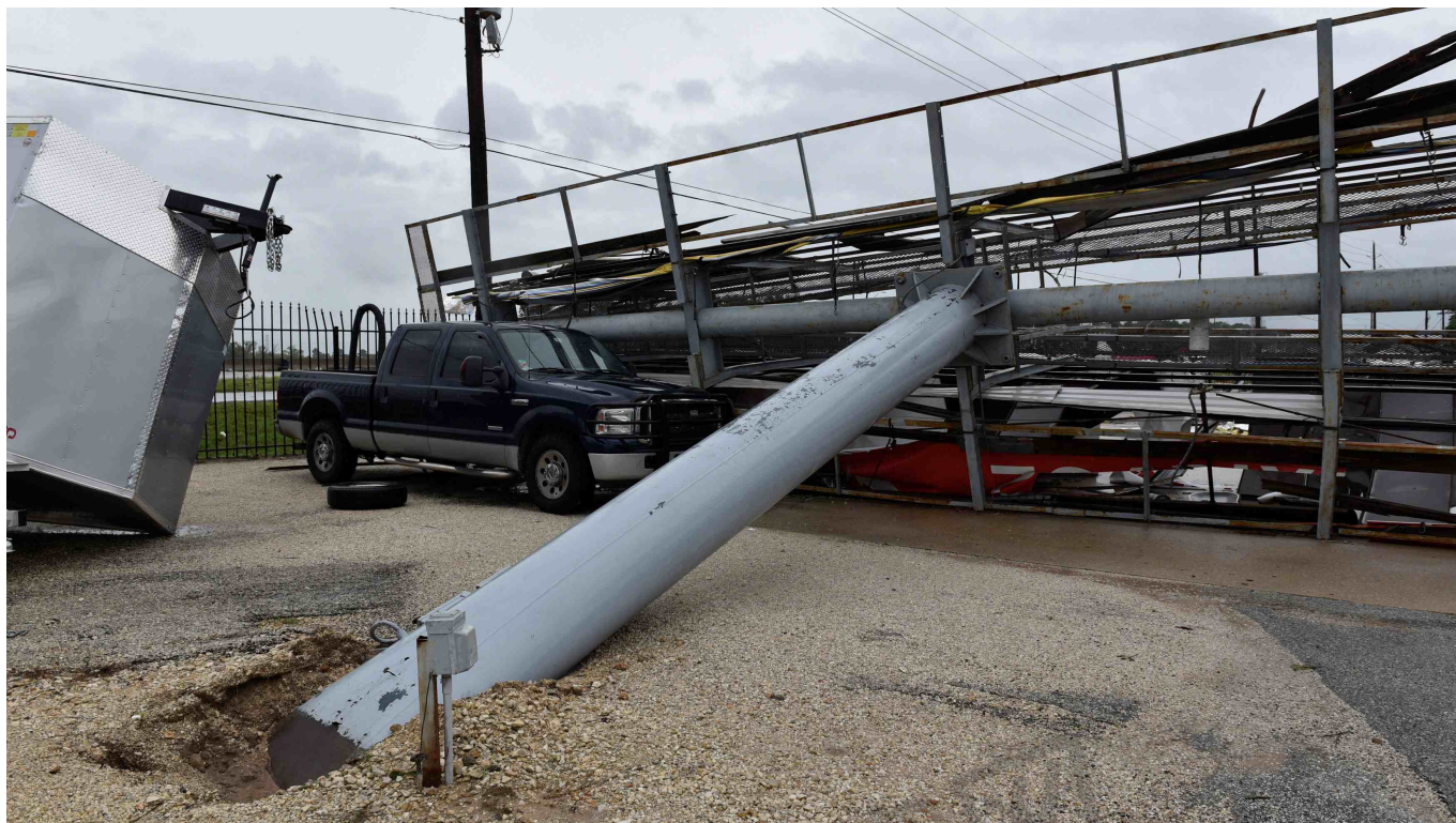
Damage left behind by a tornado that spun off of Hurricane Harvey after the storm made landfall on the Texas Gulf coast, in Katy, Texas on August 26, 2017. /Reuters Photo
