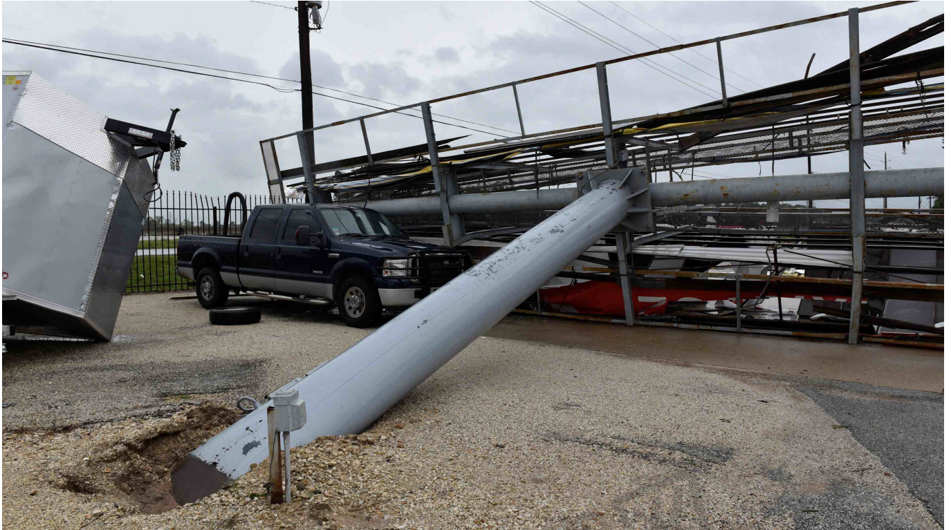
Damage left behind by a tornado that spun off of Hurricane Harvey after the storm made landfall on the Texas Gulf coast, in Katy, Texas on August 26, 2017. /Reuters Photo
