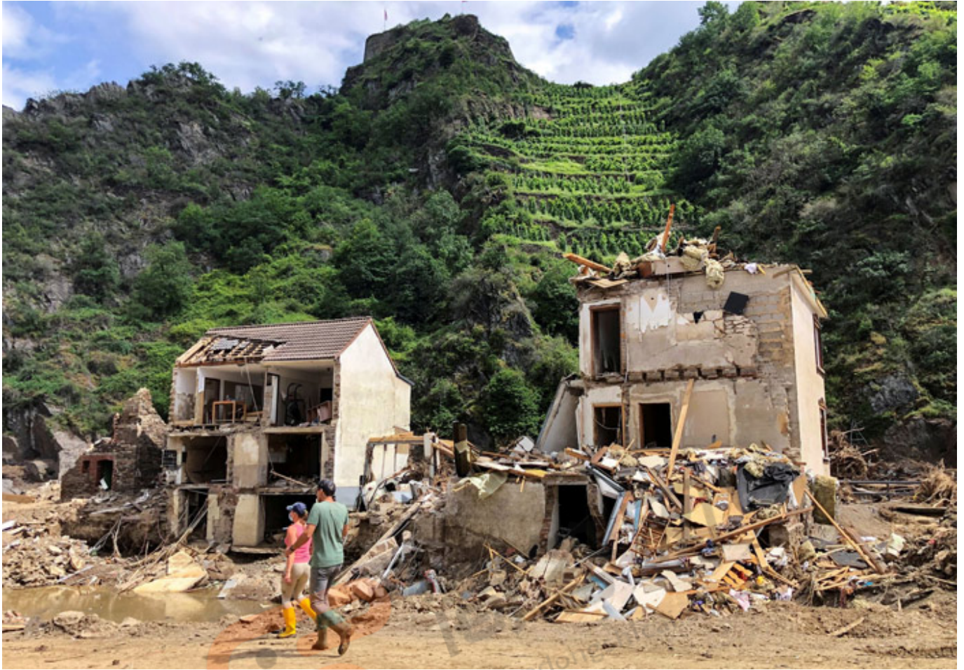
Houses destroyed by the flood are pictured in Mayschoss, Germany, July 29, 2021. REUTERS/Andreas Kranz
