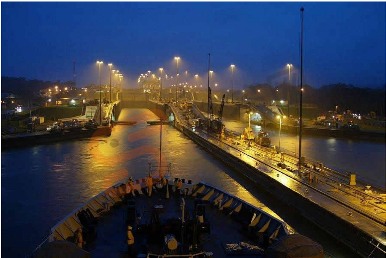
The Panama Canal. /VCG Photo
